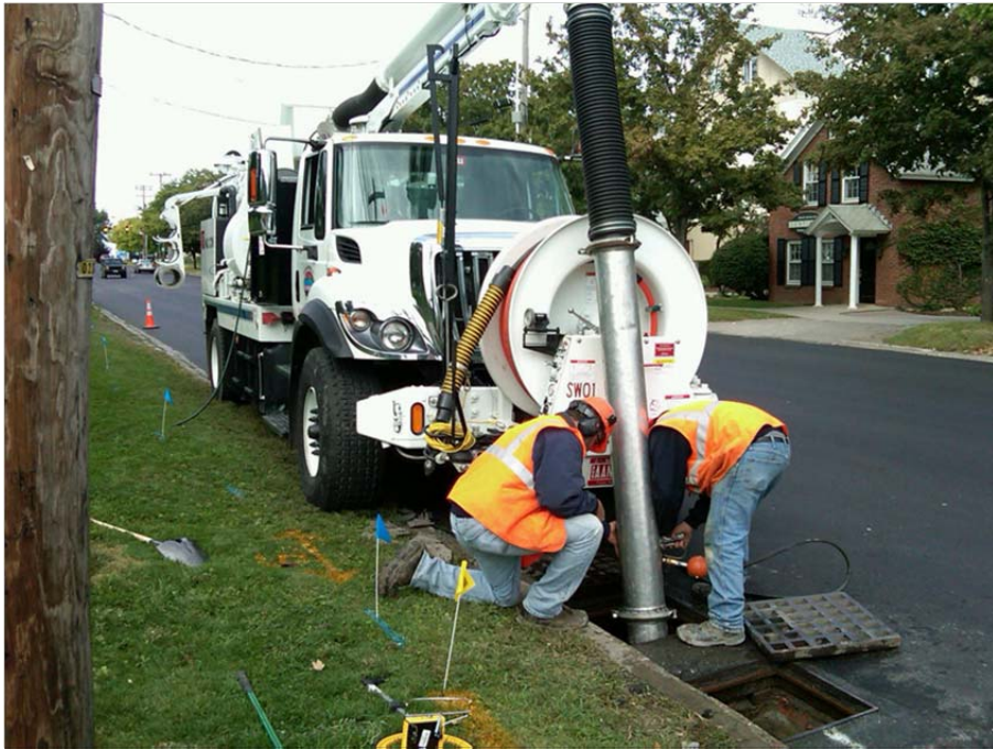
ROW employees cleaning a catch basin on Colchester Ave with the new Stormwater Vector Truck
