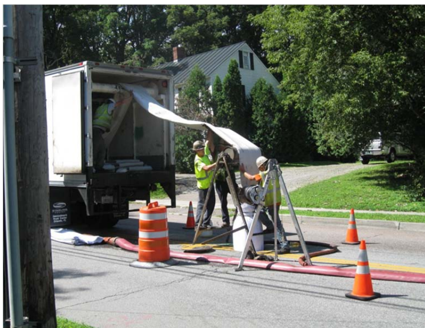
Installing of CIPP on Colchester Ave
