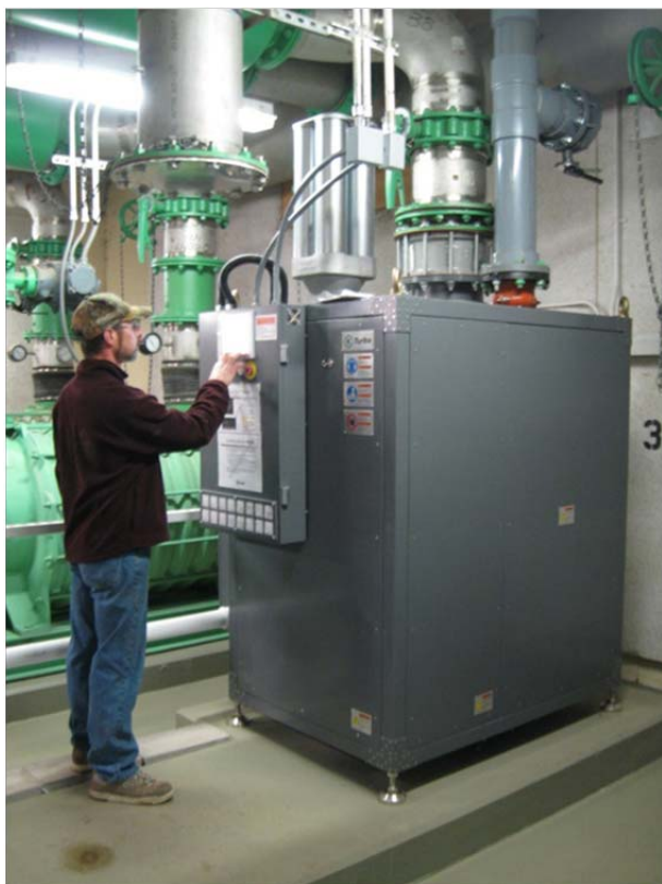
New Turbo Blower at Main Wastewater Plant
