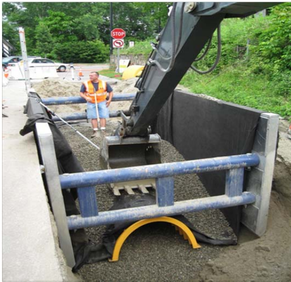
Infiltration System Installation at North Willard
