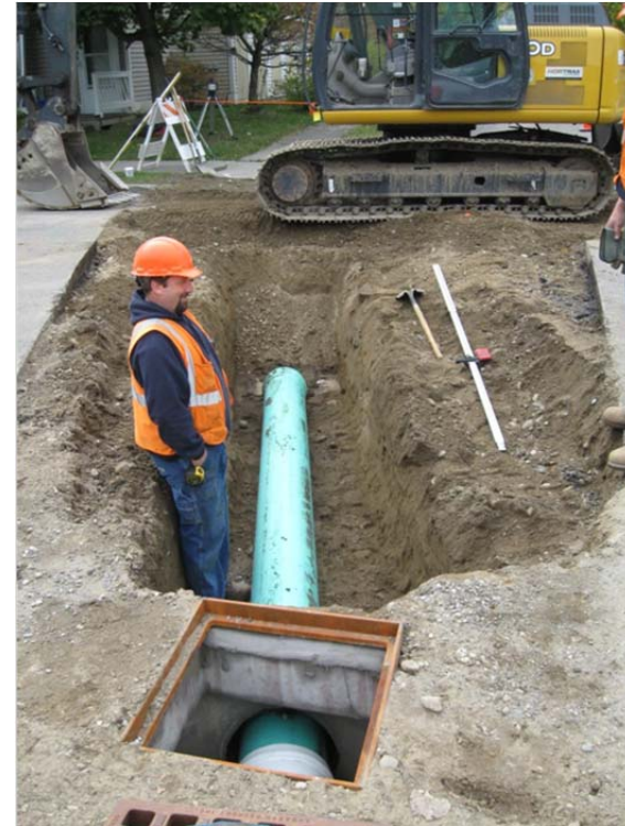
R.O.W Installing Stormwater Lines
