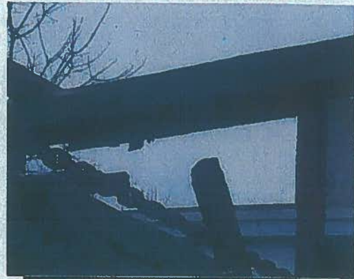
Photo D: Charred Existing Beam
